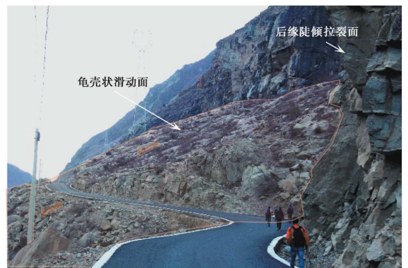
图 11 受多组结构面控制的堵江滑坡残余滑面特征 Fig. 11 Characteristics of residual slip surface of landslide dam controlled by multiple structural planes
